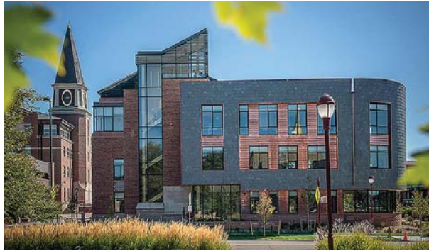
The Burwell Center for Career Achievement at the University of Denver. Credit: University of Denver
