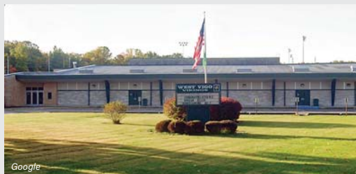
West Vigo High in West Terre Haute, Ind., is one of three high schools in the Vigo County district in line for HVAC upgrades.
