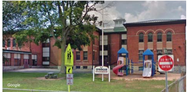
Sprague Elementary School in Waterbury, Conn. has received a $2.1 million state grant to upgrade its HVAC system.
