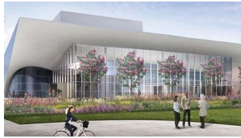
Cal State San Bernardino is constructing a $126 million performing arts center. California State University, San Bernardino
