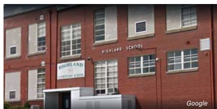
Highland Elementary School in Greenville, Tenn., has been awarded a $410,000 grant from the Tennessee Valley Authority to upgrade its HVAC system.
