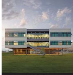
BLUE RIDGE ISD, BLUE RIDGE ELEMENTARY SCHOOL
