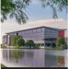
COLLEGE OF THE MAINLAND, STEAM/ ALLIED HEALTH BUILDING
