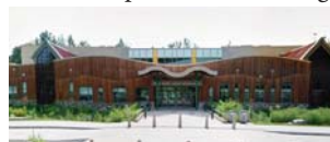
Sandy Hook Elementary School in Newtown, Conn. Image courtesy of Google
