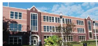
Sandels Hall at Florida State University has been closed because of the presence of mold and radon. Image courtesy of Florida State University
