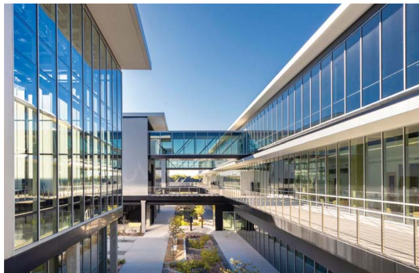
Outdoor spaces support the social life at Collin College in Allen, Texas, and create opportunities for collaboration. Image courtesy of Steinkamp Photography
