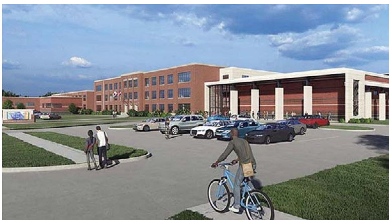
Lanphier High School in Springfield, Ill., is undergoing a $93.2 million renovation.
