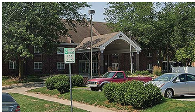
A former Holiday Inn Express in Des Moines, Iowa, will become a residence hall for Drake University. Credit: Google
