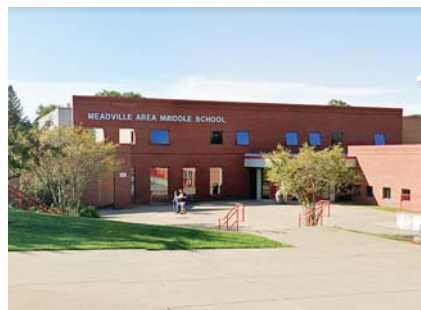
Meadville Area Middle School and Meadville Area High School have newly installed roofs.
