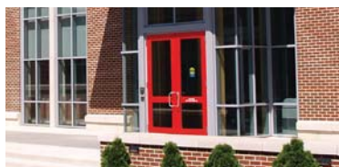
Texas officials say they will examine every exterior school door in the state to determine if security upgrades are needed.
