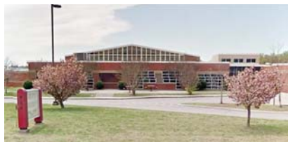
Tullahoma High School in Tullahoma, Tenn., is replacing its 65-year-old roof.
