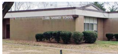
The Richmond (Va.) district is replacing part of the roof at the formerly shuttered Clark Springs Elementary School.
