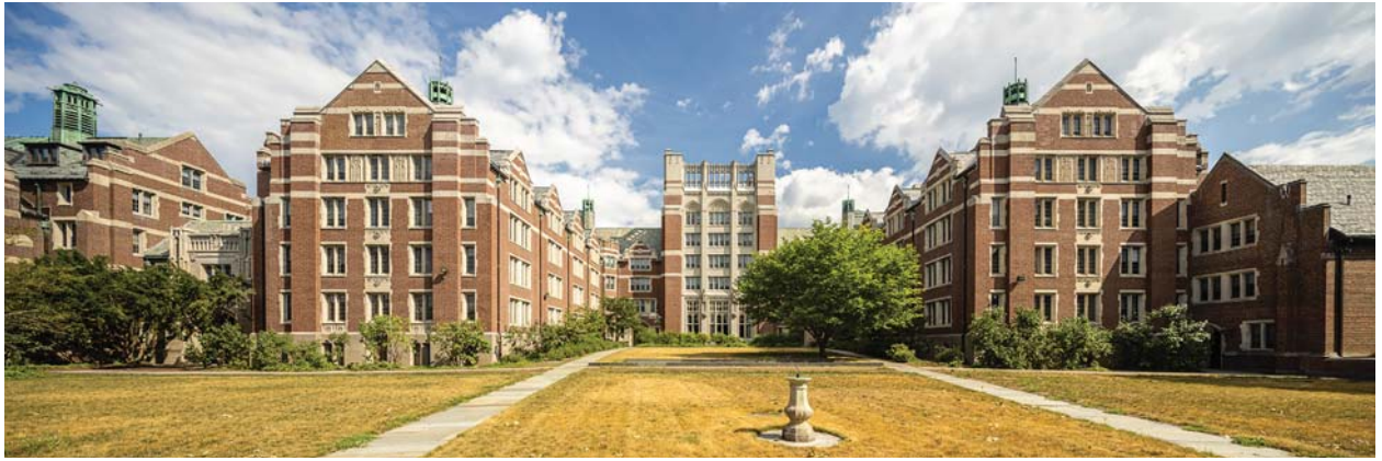
Planned upgrades at Wellesley College include converting the campus energy system from a steam distribution loop to low temperature hot water.
