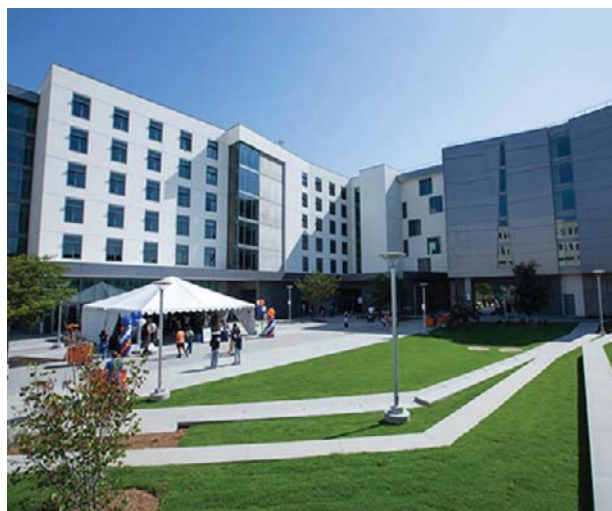
A suite-style residential community for 600 students has opened at Cal State Fullerton. Image courtesy of California State University, Fullerton.
